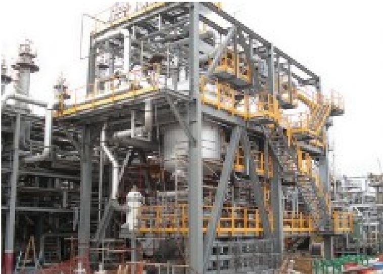
**August, 2006 - Greece:** Hellenic Petroleum S.A. awards Siirtec Nigi a contract for the engineering, procurement and construction of a Sulfreeen tail gas treating unit on the Thessaloniki project. The plant is designed to increase the sulphur recovery of the existing sulphur plant from 96% to 99%. The technology package for this sub dew point process was supplied by Lurgi.
